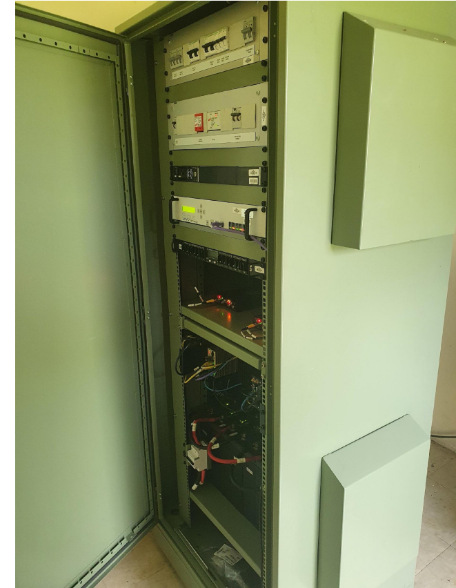
Instrument rack – GNSS Hut
