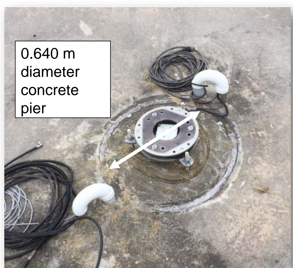
Existing concrete pad surrounds two piers going to 6' depth
