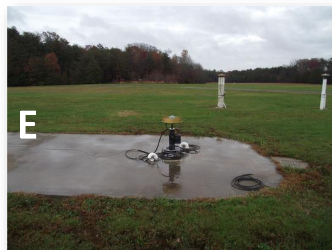
Existing concrete pad surrounds two piers going to 6' depth
