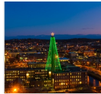
Wanalancit Building Lowell, Dec 2015 Home to Digisonde®
