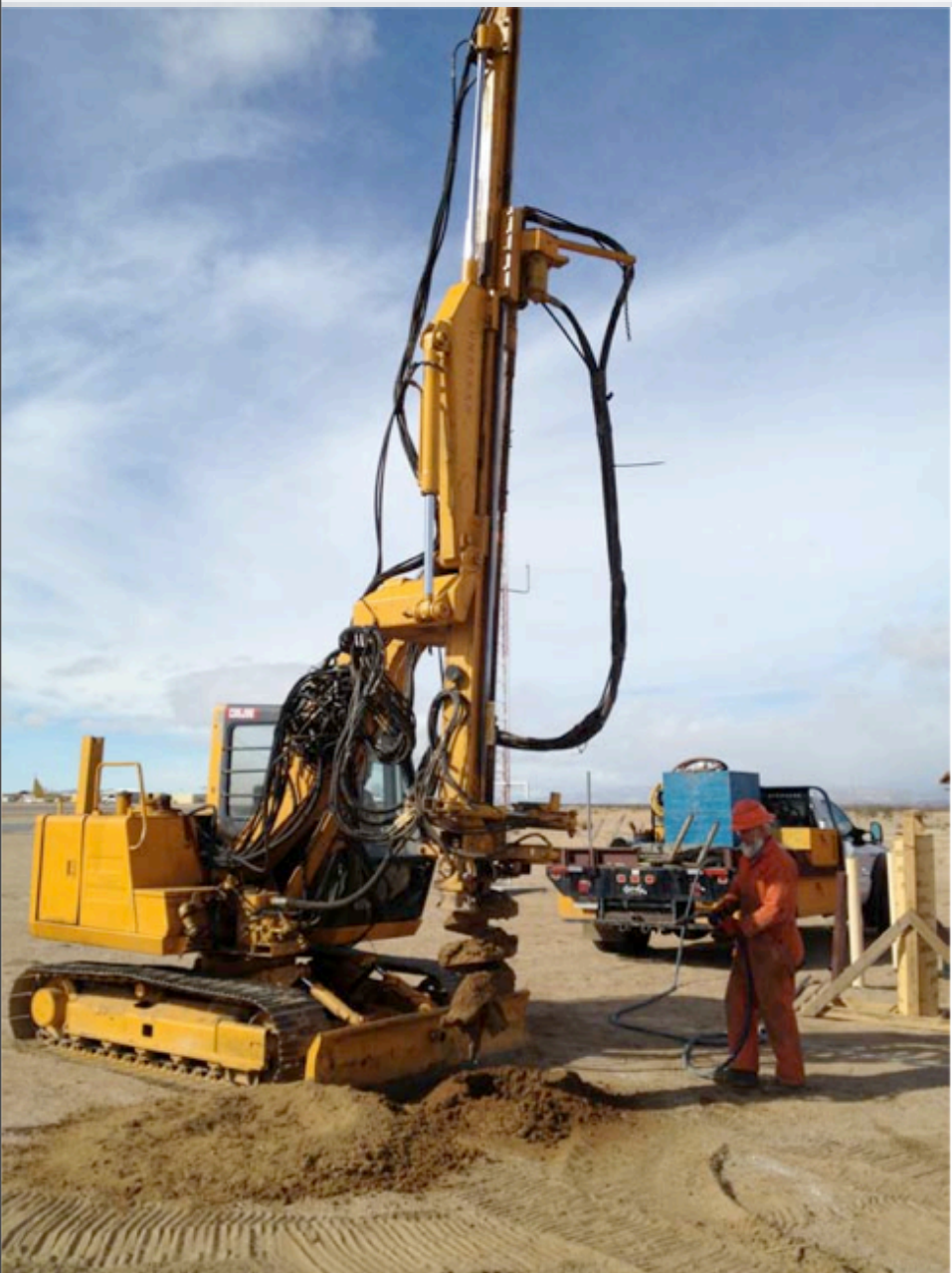
18" diameter hole about 15ft deep
