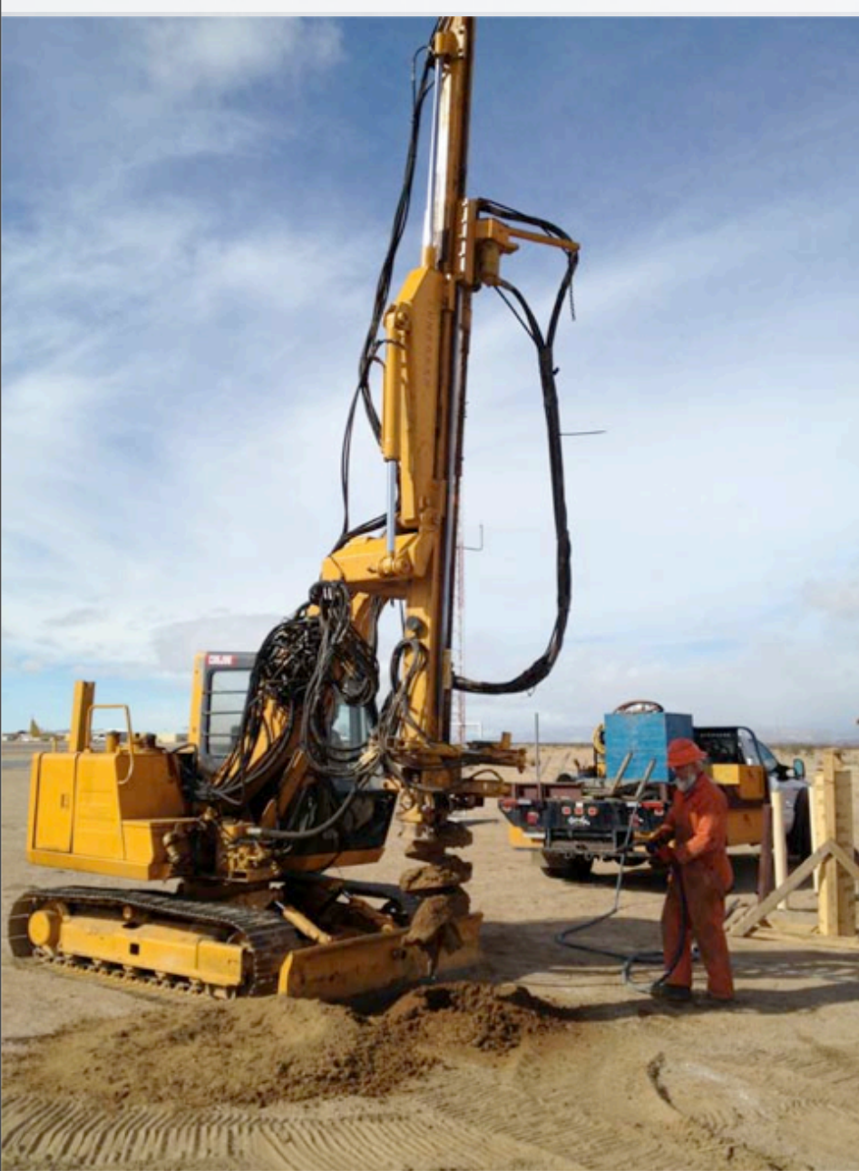
18" diameter hole about 15ft deep
