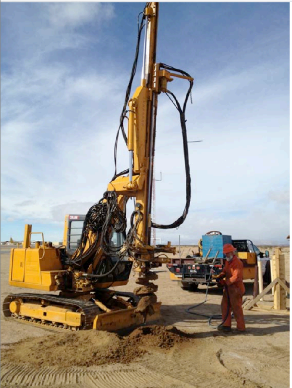
18" diameter hole about 15ft deep
