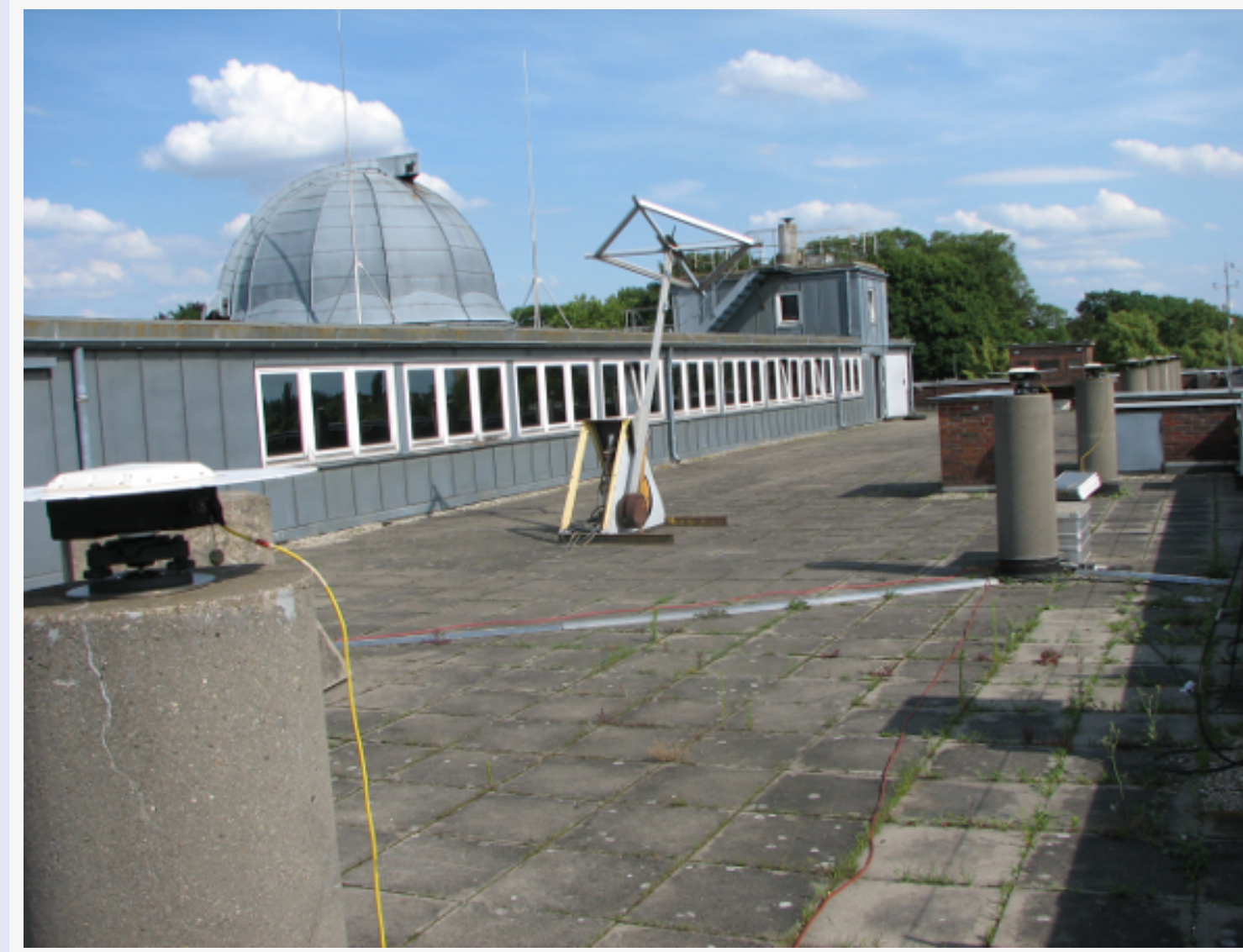
Fig. 1: Laboratory Network at the rooftop.
